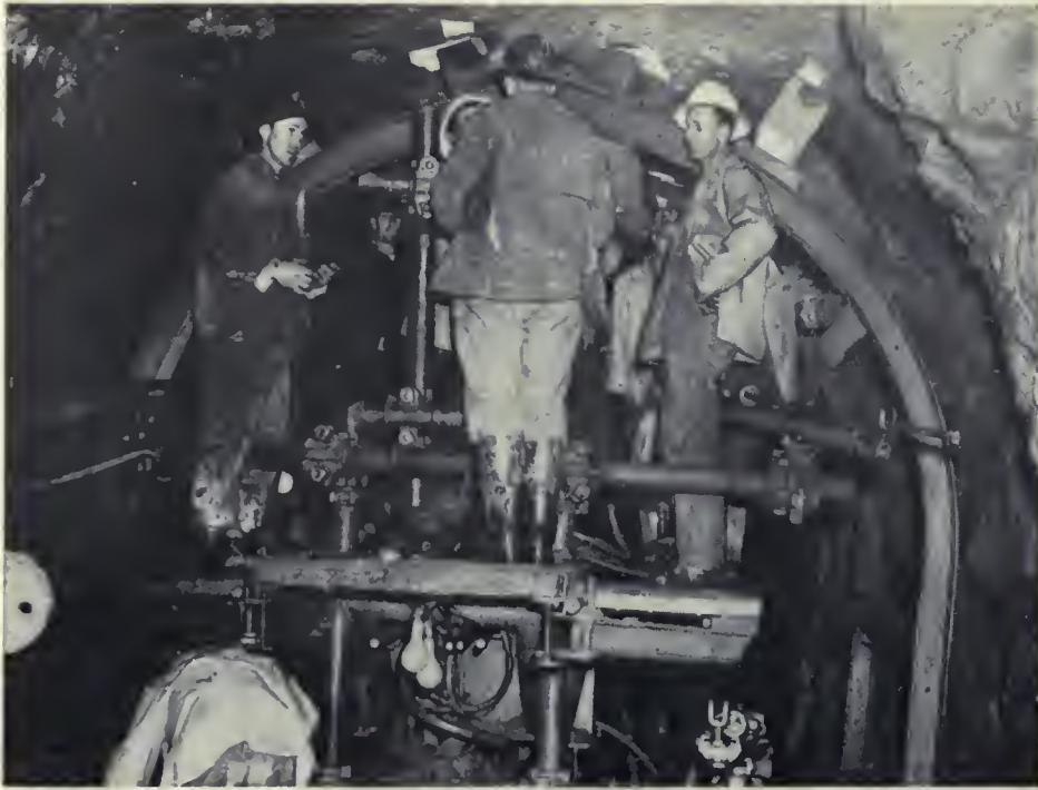
TROUBLESOME TUNNEL— Above, jumbo set-up for drilling in tight spots to install steel supports. Above right, workers' "Subway." Center right, checking the roof. Immediate right, reconditioned tunnel. Next, "Diogram for Destruction." "Diogram" photo by W. Broodfoot, Region 4, "Subway" photo, photographer unknown, others by M. F. Edwards, Region 4.
